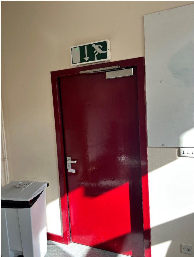
Front of LT access and emergency egress door
