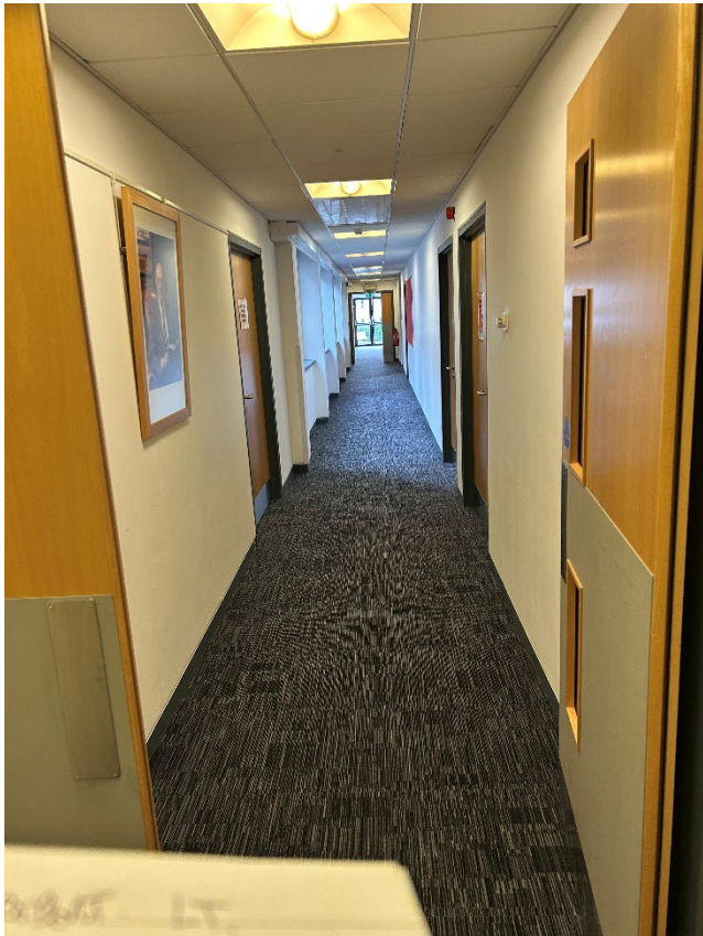
Escape door at the end of the corridor
