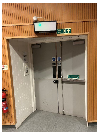
Emergency exit door at the front of LT
