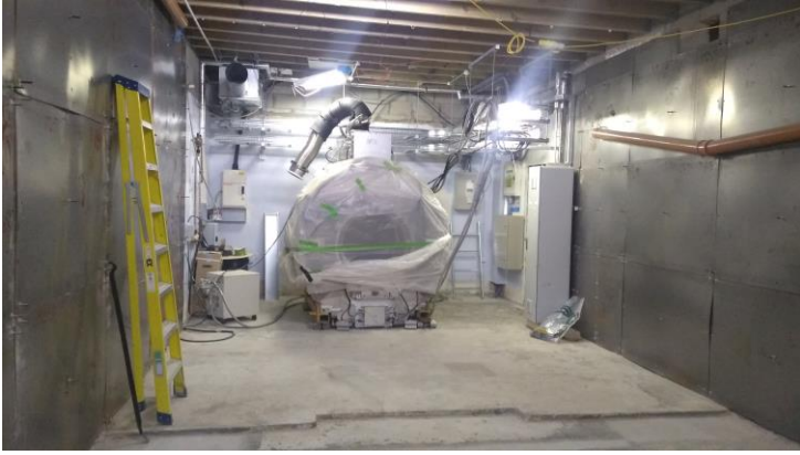
Scan room after the RF cage has been removed with a close-up of the “roller skates” used so the magnet can be moved around the room.
