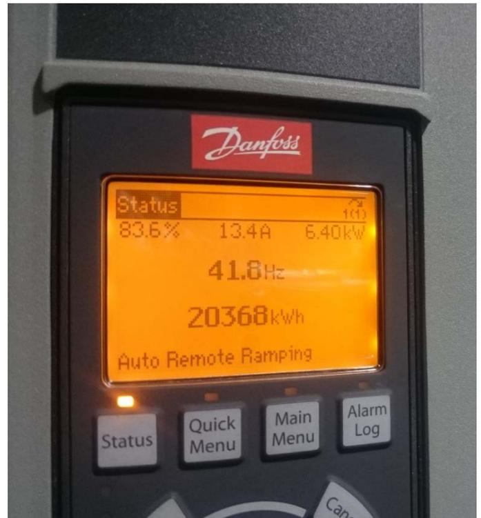
Pump Speed and Consumption after VSD Installation
