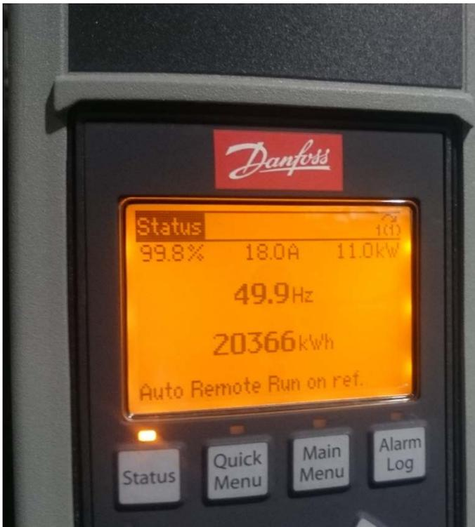
Pump Speed and Consumption before VSD Installation
