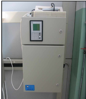
Fig. 1. Loop Flow Analyzer
