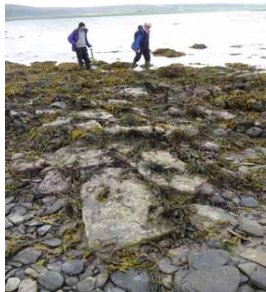
Figure 19: Jetty at Ferry Point
